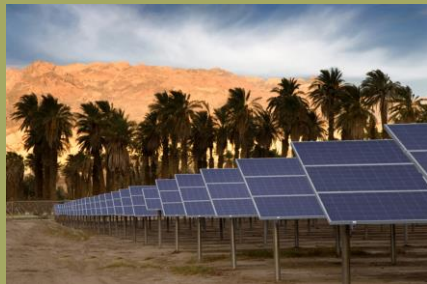
A five-acre, 1.23 megawatt solar photovoltaic system generates 2.3 million kWh per year, enough to power more than one-third of the total annual electricity needs of Xanterra's Death Valley operations.
