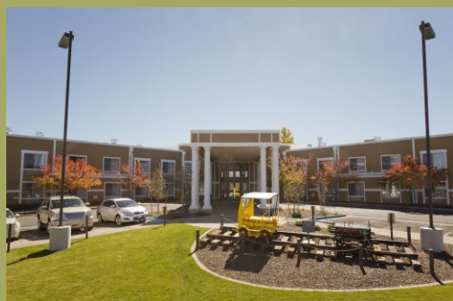
Grand Canyon Railway Hotel has reduced natural gas consumption by 17 percent.
